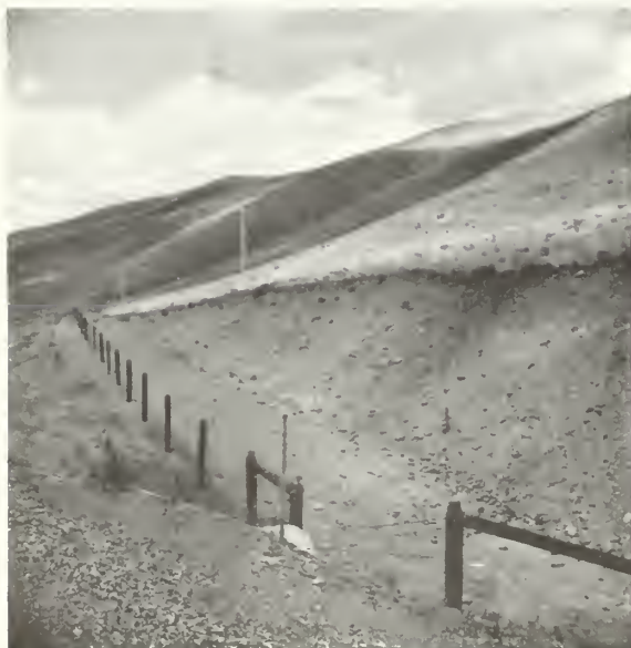
East approach to underpass
